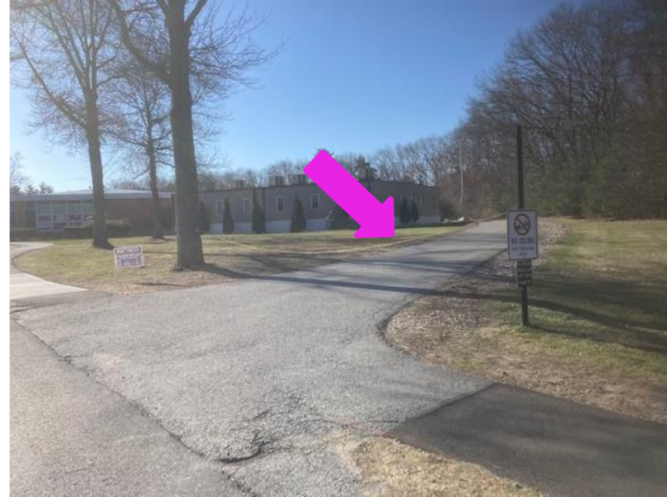
The entrance to the school's rear driveway at Westwood Street uses a rope to bar entrance during school hours. There is no crosswalk or identifying signage.
