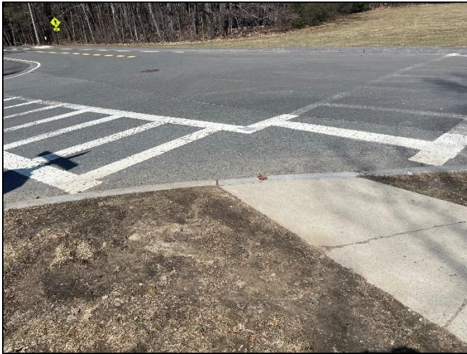
Photo 15: Accessible ramps lack detectable warning panels throughout the study area.
