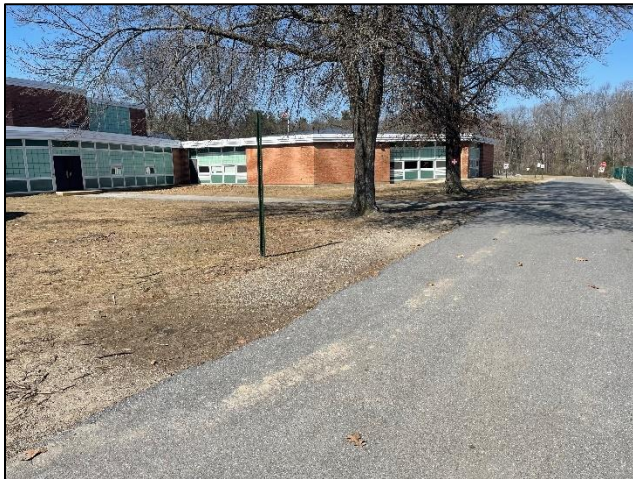
Photo 7: Parent vehicles unload at the east side of the building and students enter through the side doorway.
