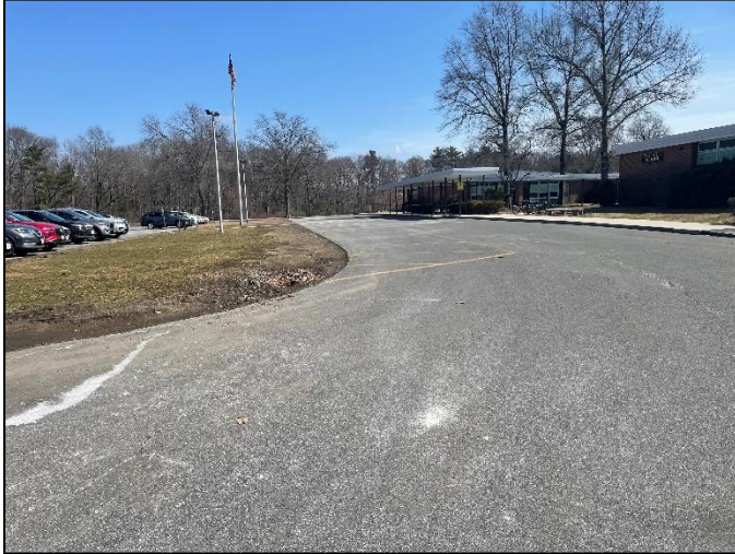
Photo 1: The front of Fox Hill Elementary School is used for bus drop-off/pick-up operations.
