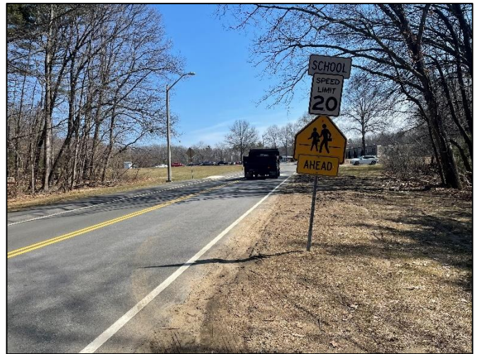
Photo 18: School speed limit sign assemblies do not align with current standards.
