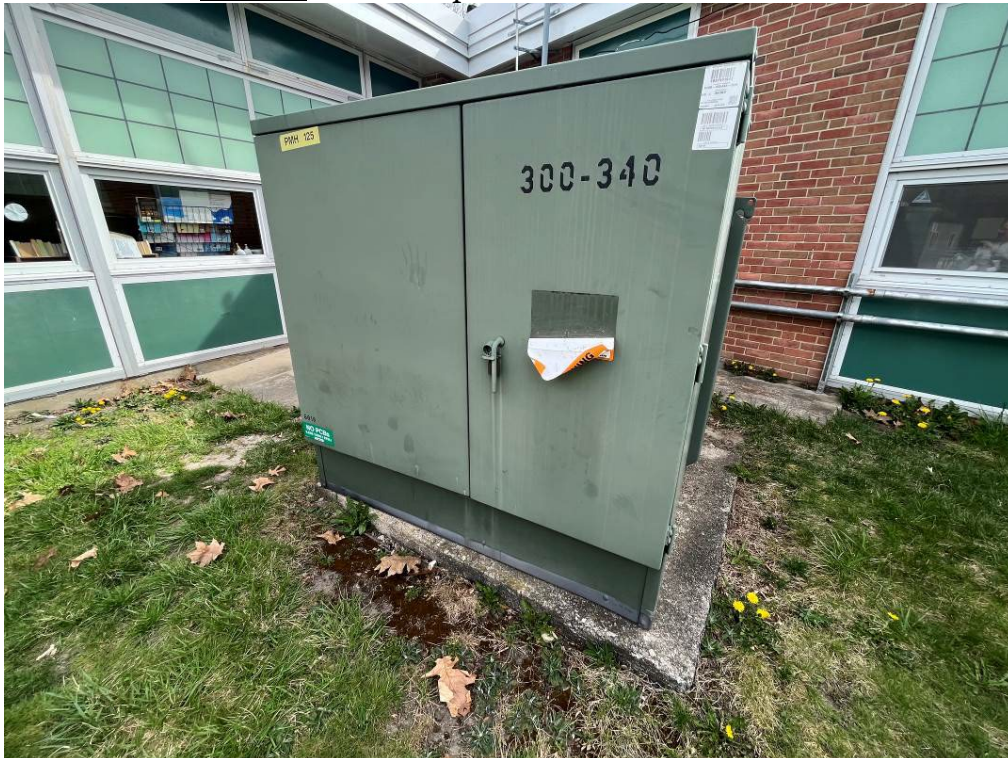
Photo 6 – View of pad-mounted transformer.
